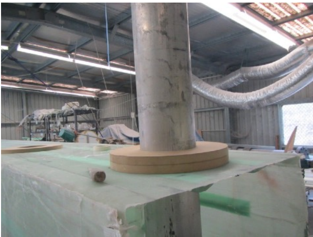
MDF will create lands to support the mast
